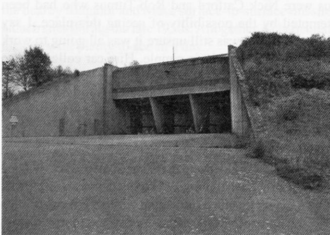
Typical vehicular entrance to a shelter.
